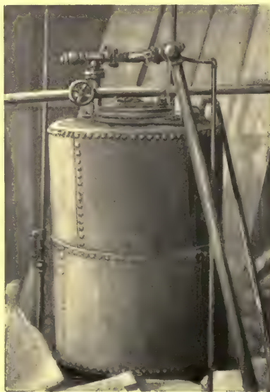
FIVE-BARREL STILL USED IN THE FIFTIES IN DISTILLING CRUDE OIL AS A LUMINANT
